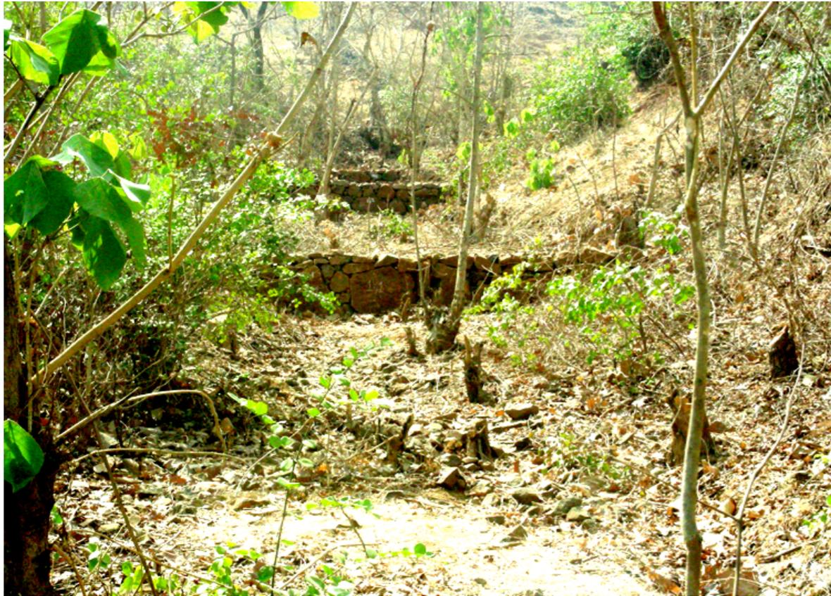
*'Gully Plugs' ( mini-dams of boulders) to hold back top-soil & water at each contour level of hill slopes.*
